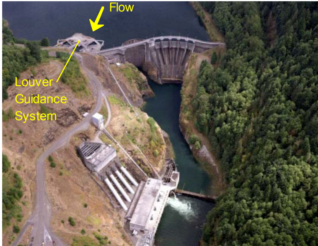
Figure 3-27. Aerial photo of Mayfield Dam
