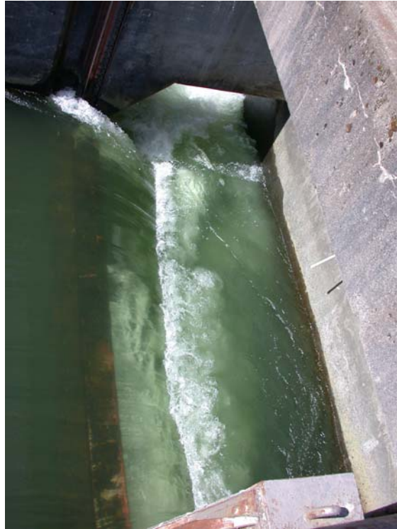
Single Entrance to Ice and Trash Sluiceway: Currently in use
