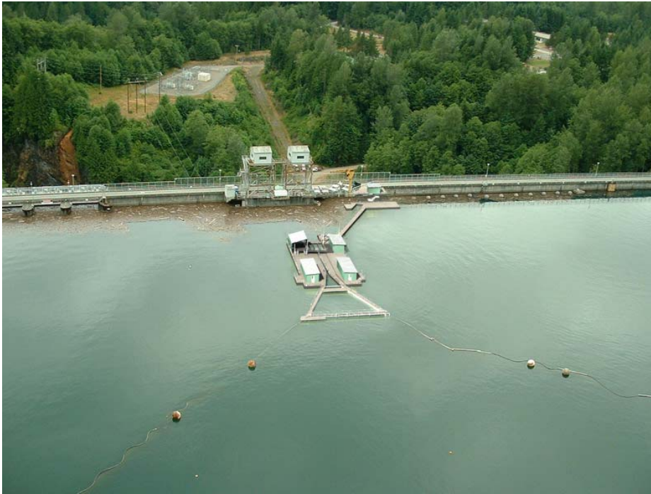
Figure 4. Upper Baker forebay aerial showing rendering of future FSC, NTS and net.
