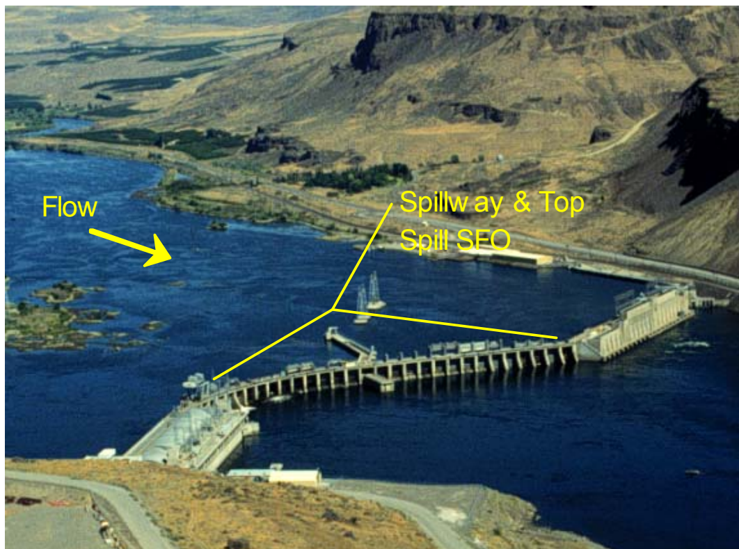
Figure 3-5. Aerial photo of Rock Island Dam
