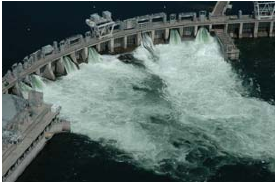
Figure 3-6. Top spill at Rock Island Dam
